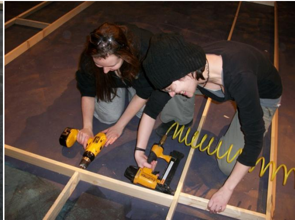
Constructing the Set
